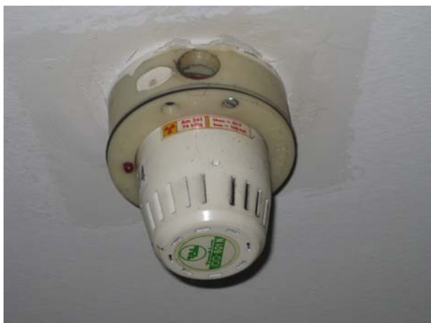
Figure 19: A smoke detector with ^{241}\text{Am} of 74kBq located on the ceiling of a building in downtown Ljubljana
